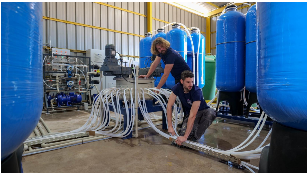
Figure 5: Puritech technicians on site during the construction phase – late December 2023
