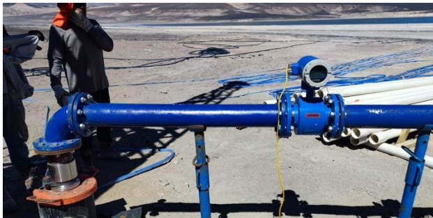
Pump test trial underway at Laguna Verde
